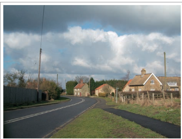
Undergrounding overhead powerlines – before
