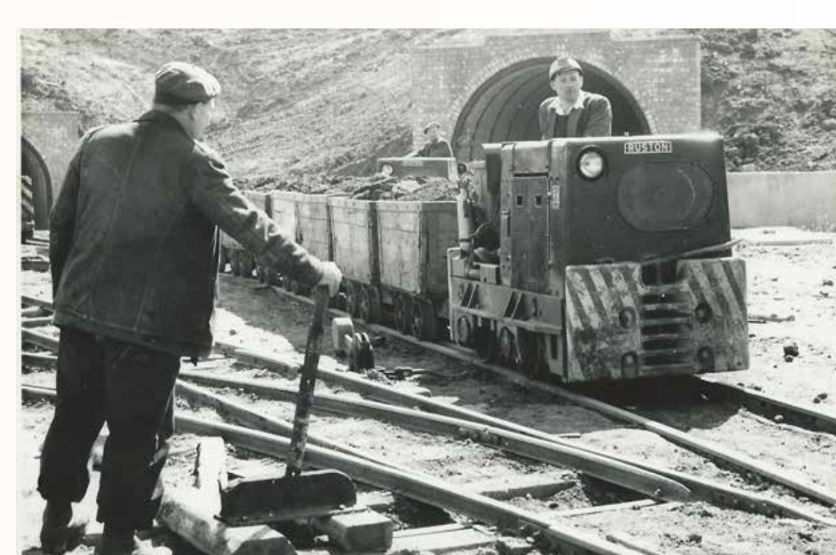
A train of ironstone coming out of the mine
