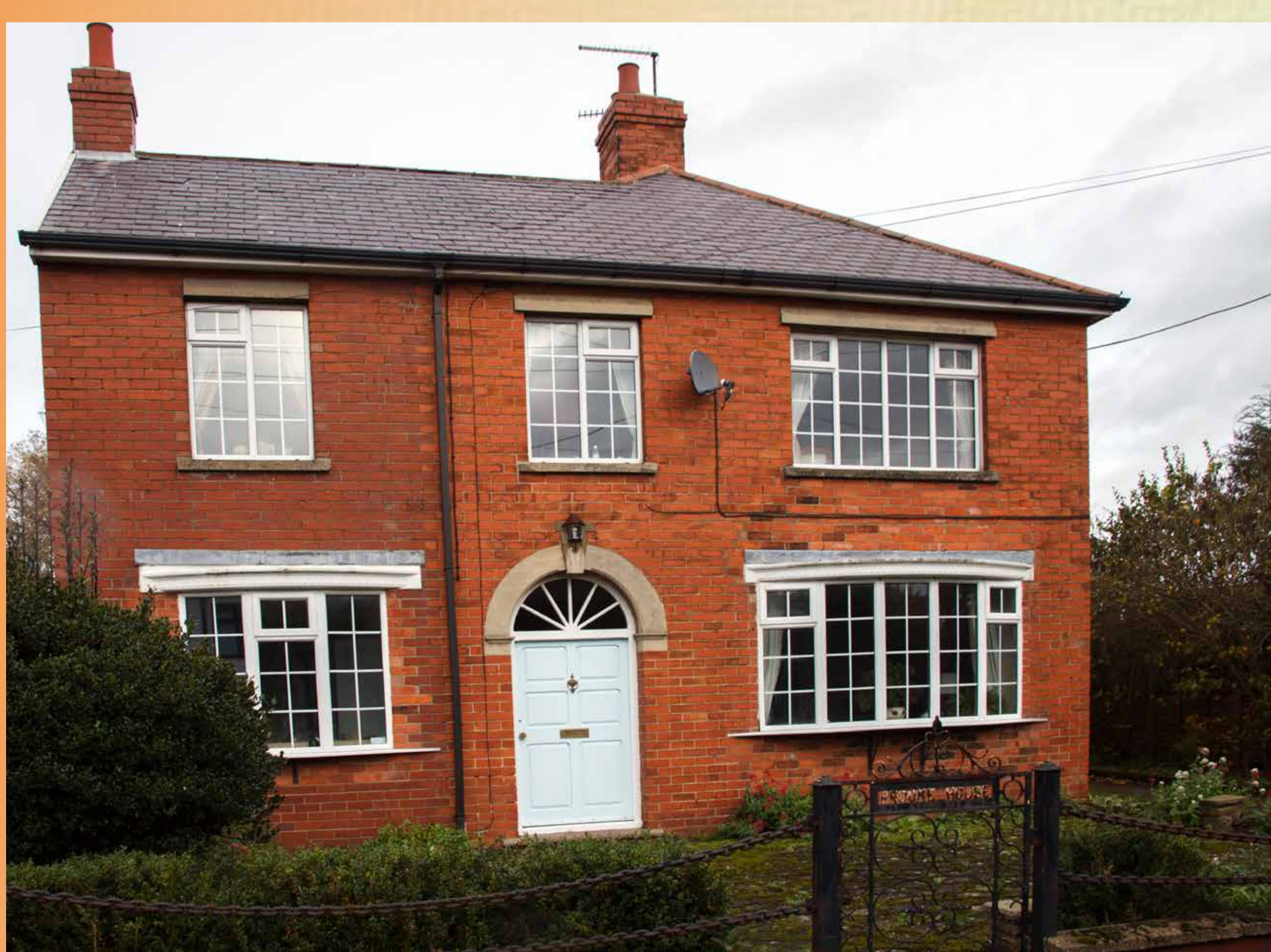
The mine manager's house in Cook's Lane
