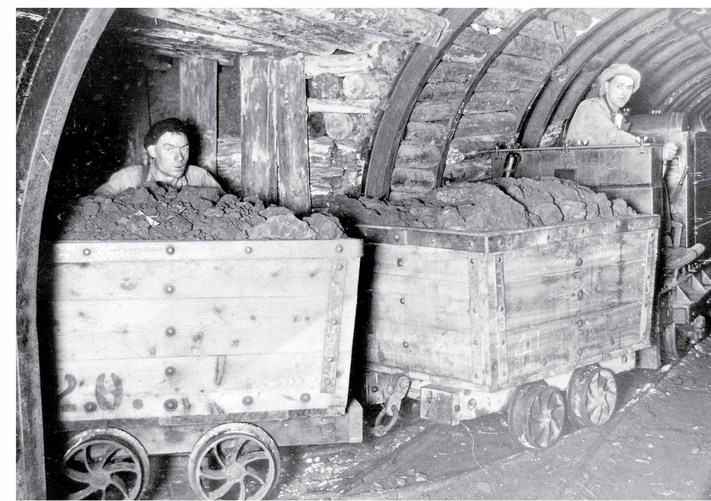
Inside Nettleton Top Mine, soon after opening, a loaded train is being taken to the surface
