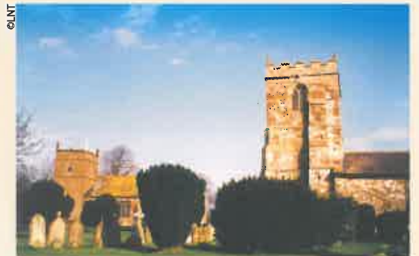
St Mary's (left) and St Adelwold's at Alvingham
